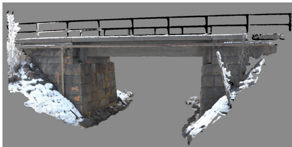
Photo of a bridge and digitalized model from photogrammetry
