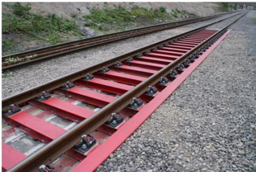
Figure 12.6b: Ladder track for improved plain line track support stiffness
